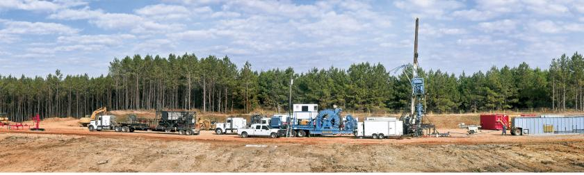
Work pregresses at a \$34 million Department of Energy funded research project evalutaing sequestration and monitoring strategies for long-term storage of carbon dioxide at Cranfield field in Mississippi. Here, an observation well is being drilled and fiberglass casing is waiting to be inserted and cemented inside the well.
