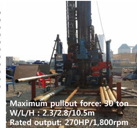
[5] Drilling of injection well and well completion
