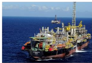
2025: 80Mt CO 2 stored in the pre-salt CCUS-EOR project
