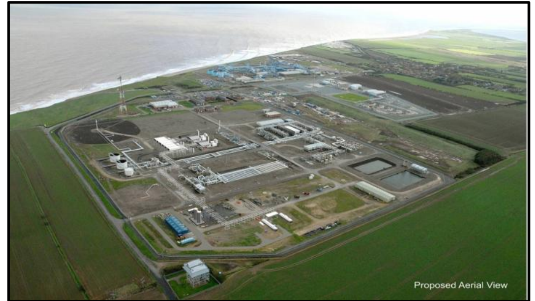
Terminal Dimlington – Capacity ~500 mmscf/d
