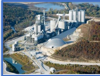
Holcim Ste. Genevieve Cement Plant Bloomsdale, Missouri
